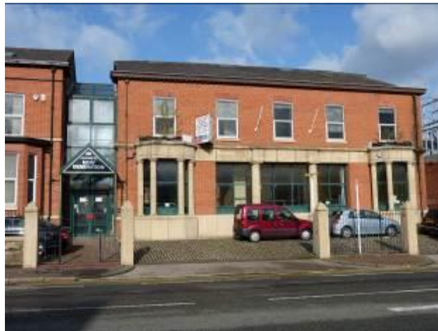
Chester Road shopfront style window, which continues the architectural balance of the adjoining terrace but which has become quite dated
