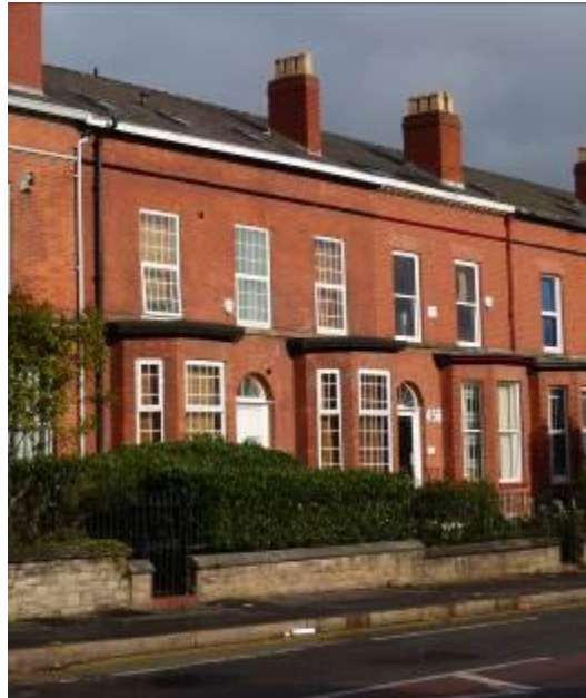
Inappropriate Georgian-style windows on the left
