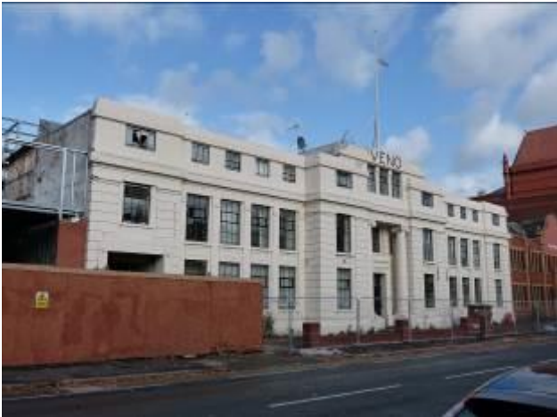
The partially refurbished Veno building; note the new windows which have been broken
