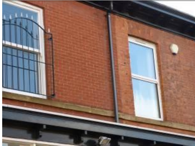
Historic Flemish bond brickwork meeting modern stretcher bond brickwork
